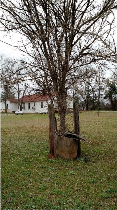
Abandoned groundwater wells are a *threat to well water, the aquifer, and public health and safety*. Abandoned wells are a direct conduit for contaminants to pollute the aquifer. Some of these contaminants can be chemical such as dumping oil, paint, or other trash into the well. Other contaminants can be bacteriological such as decaying organic matter that can leave the person consuming the water ill.
